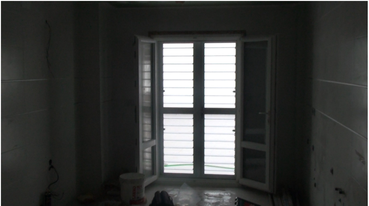
Example of the passing of light with the system of shutters in opened position and the rest closed
