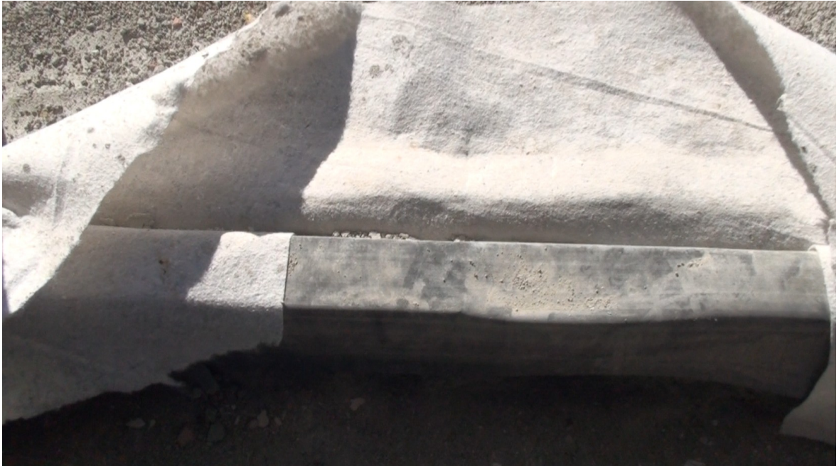
geotextile lamina to protect insulation and impermeabilisation
