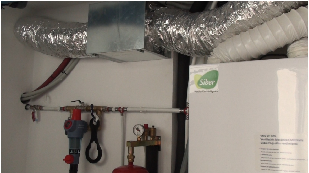
Flooding of water through the filter Honeywell FK 72CS to protect the installation from impurities
