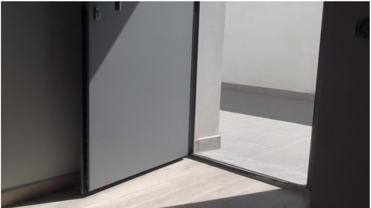
Door Hörmann TermoPro, model TPS 010 with transmittance u=1,2 \text{ W/m}^{20}\text{C}
