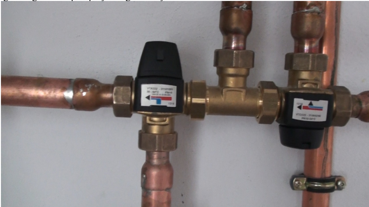
Thermostatically mix valves and selectors for solar benefits, ESBE VMC 322
