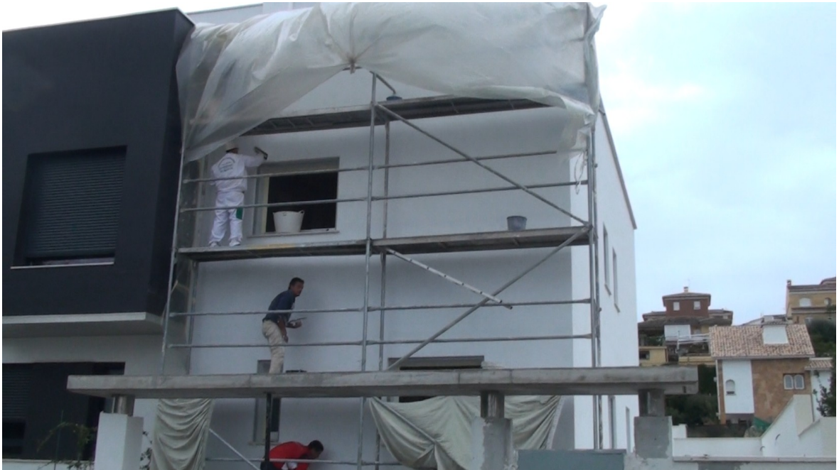
Finishing works on the ultimate layers of the facade
