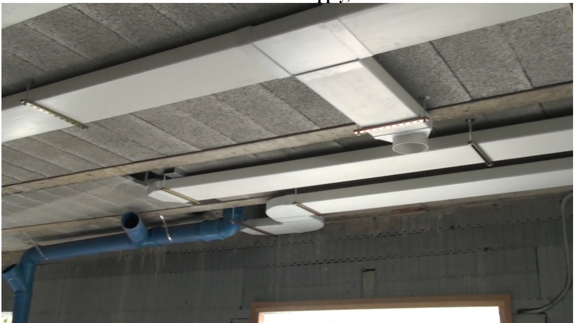
General tubes of supply, extraction and distribution of air
