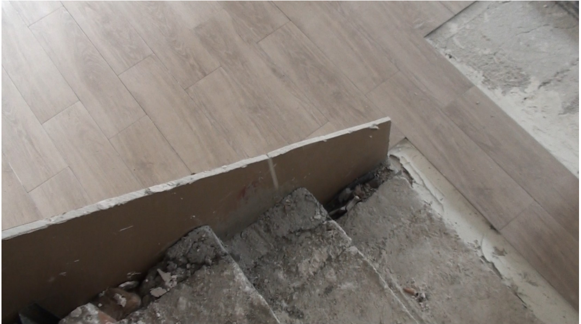
Finishing the floor with porcelain tiles looking like wood
