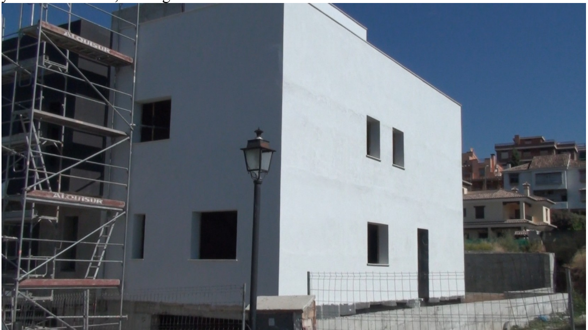
Aspect of the first three layers after removing the scaffolding
