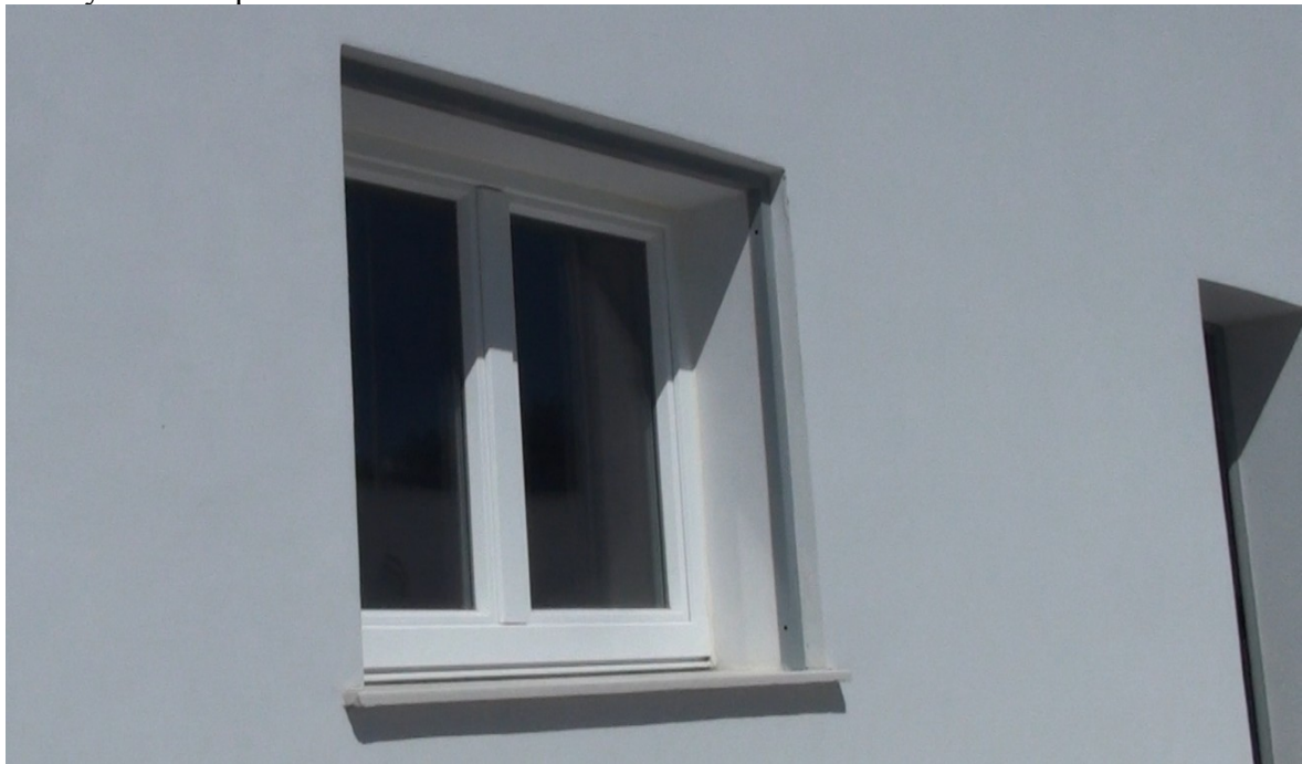
Detail of the preframe of blinds before the instalation
