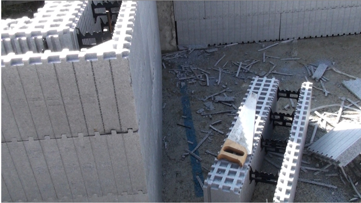
Day 1 , 19.04.2011, Setting of the first 4 layers before vertical orientation.
