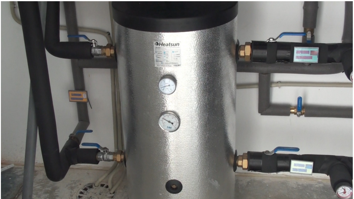
Inert deposit of floor heating
