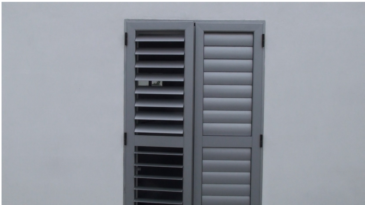
Example of different grades of opening of the louvres in a shutter
