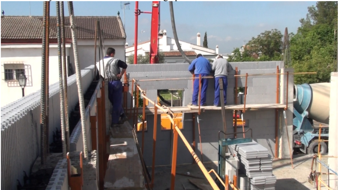
Day 3 25.04.2014 filling of the formwork until its complete height
