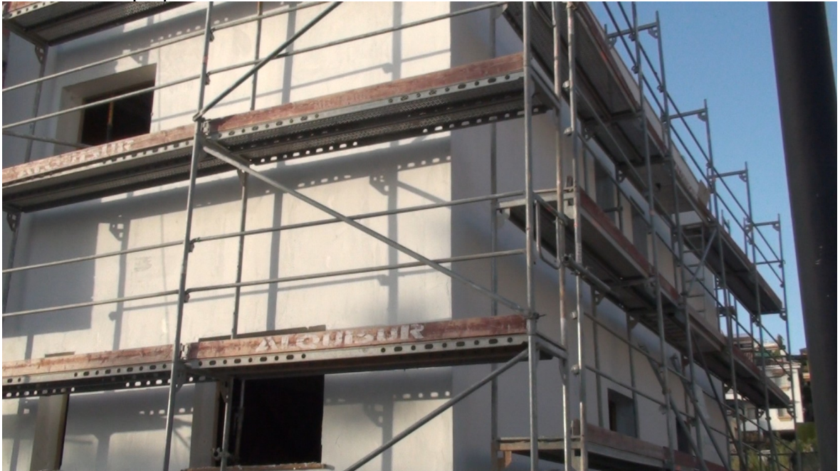
First layer of rendering to protect the insulation against ultra-violet radiation.
