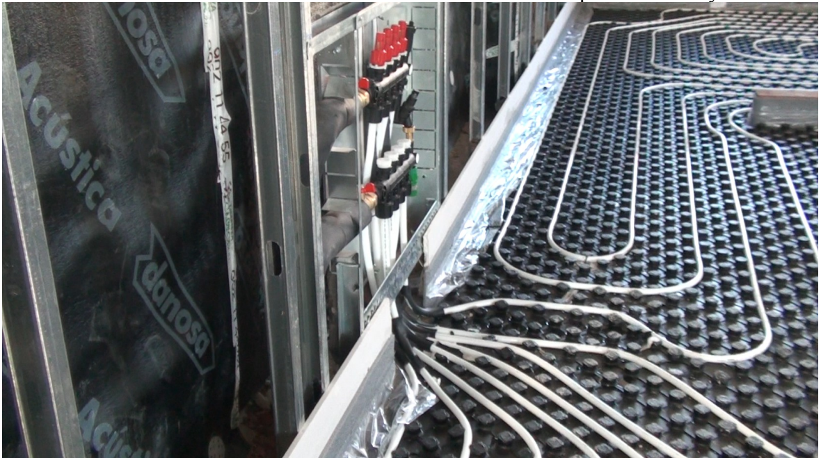
Low temperature heating system in floor heating of the brand Uponor
