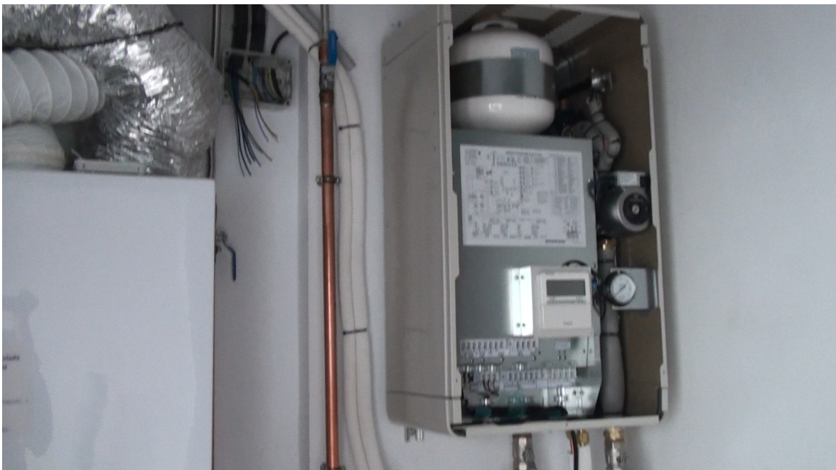
Internal unit of interchanging boards of the system Estia
