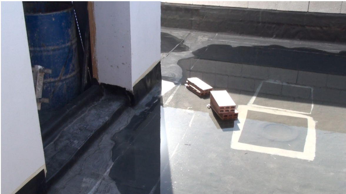
waterproofing with EPDM by Firestone, much better than bituminous membrane
