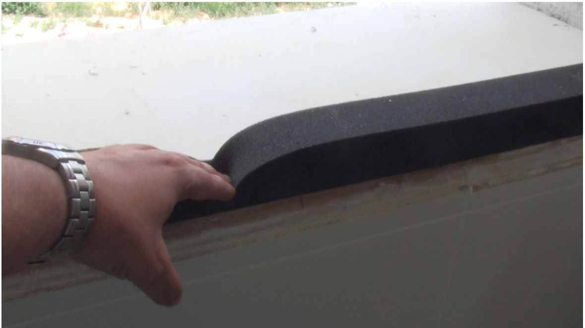
Detail of the material that supports the frame of the window to a perfect fit
