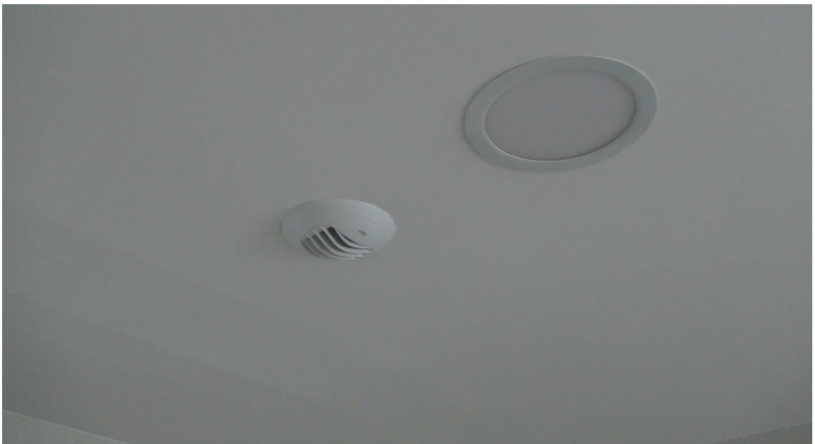
Extraction mouth for stale air together with the LED in the ceiling
