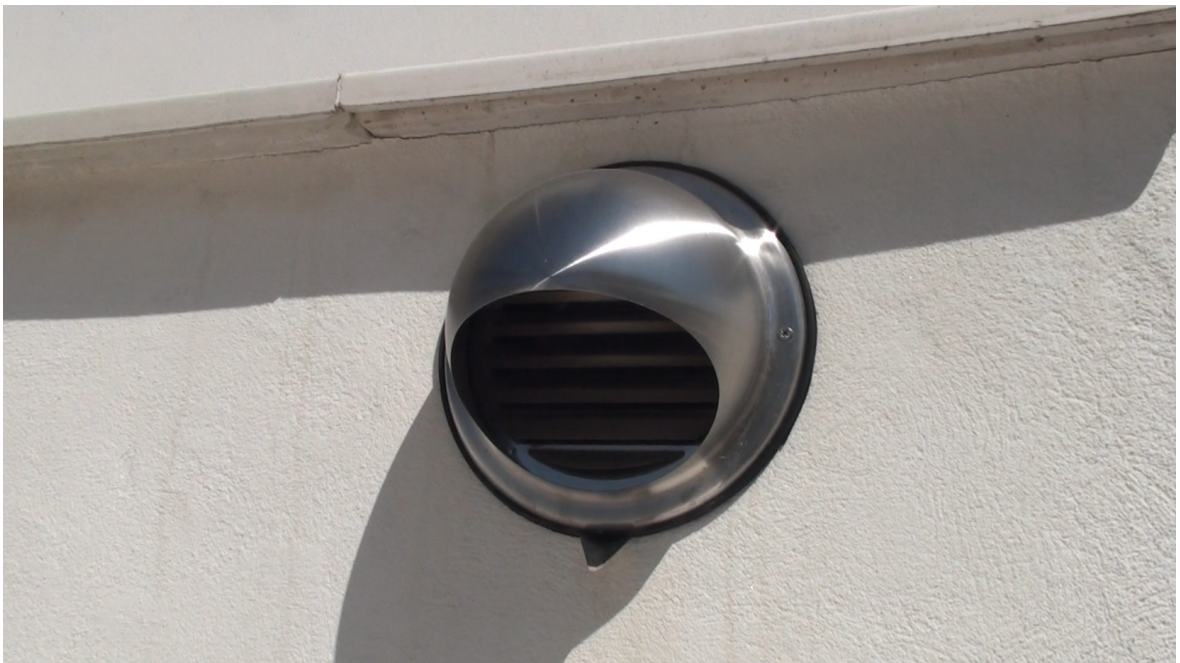
Detail of the mouth for fresh air to the interior of the house
