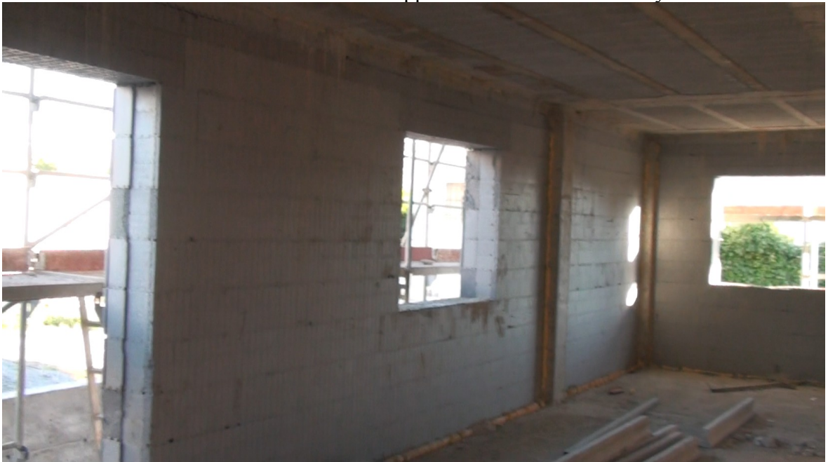
Following days – finishing of gaps for windows and doors
