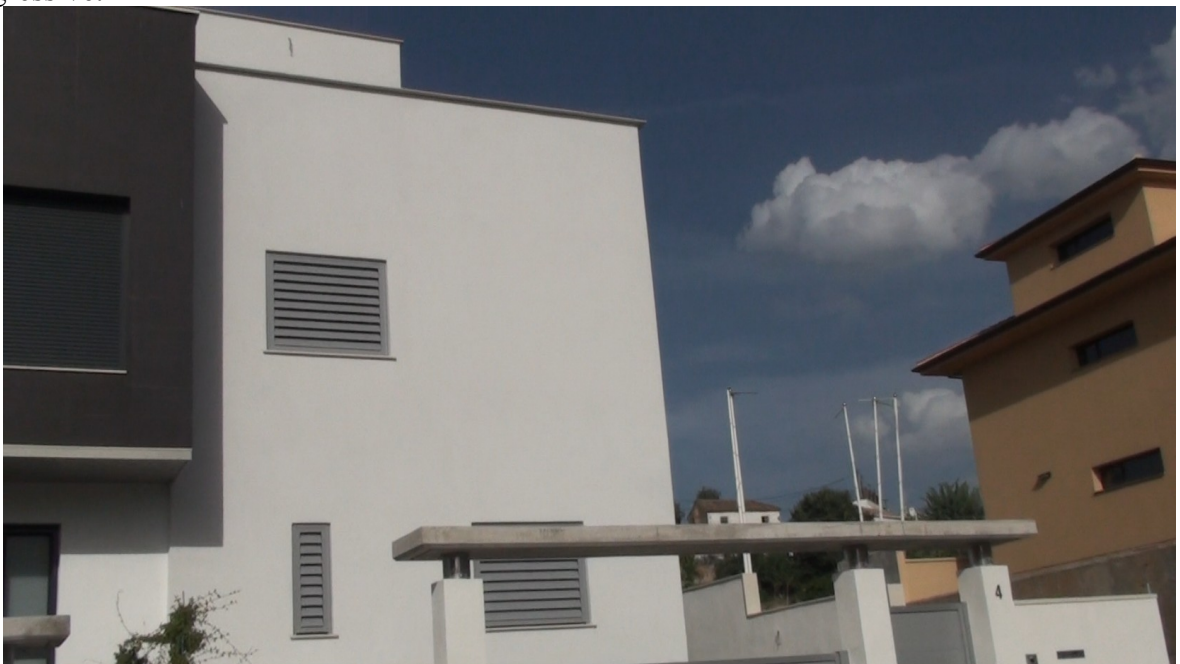
View of the facade with the coating finished
