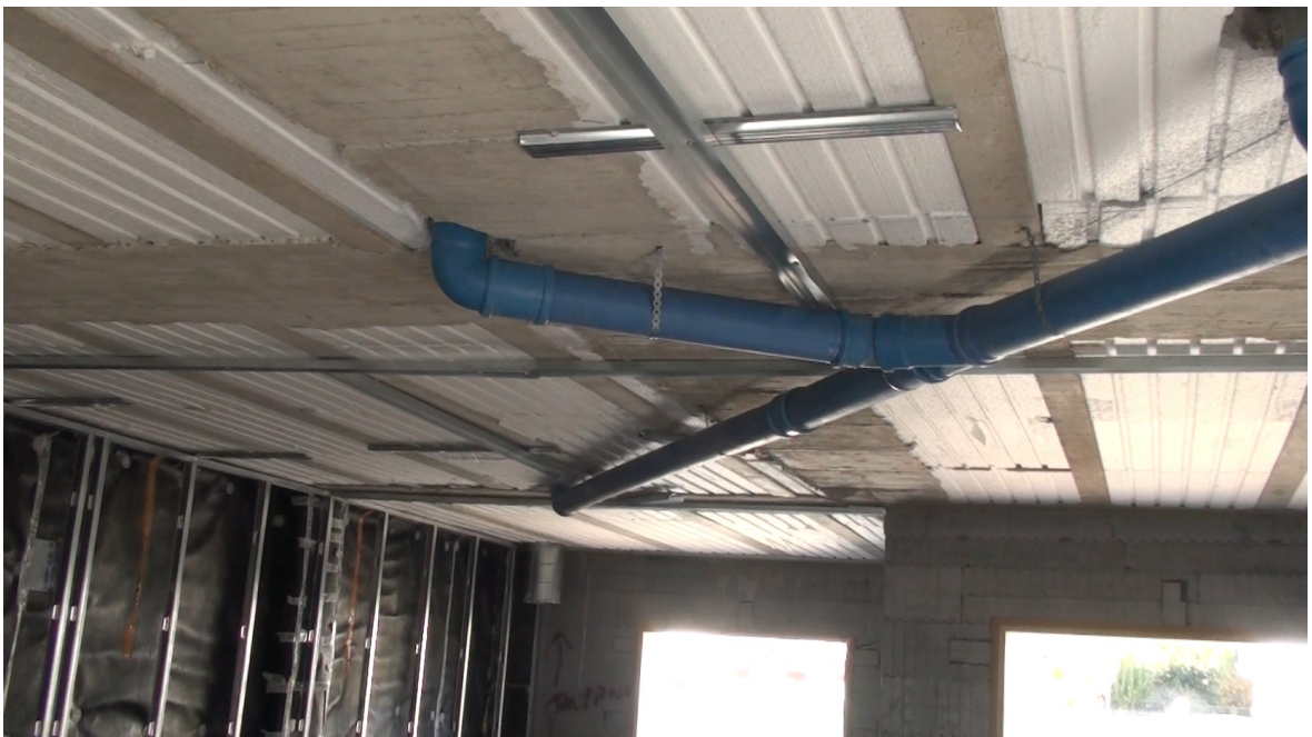
Insulating floor blocks in the ceiling of the last floor
