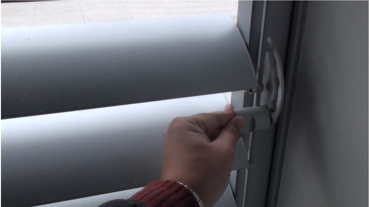
Example of the manual regulation which allows inclinations inverse above the horizontal
