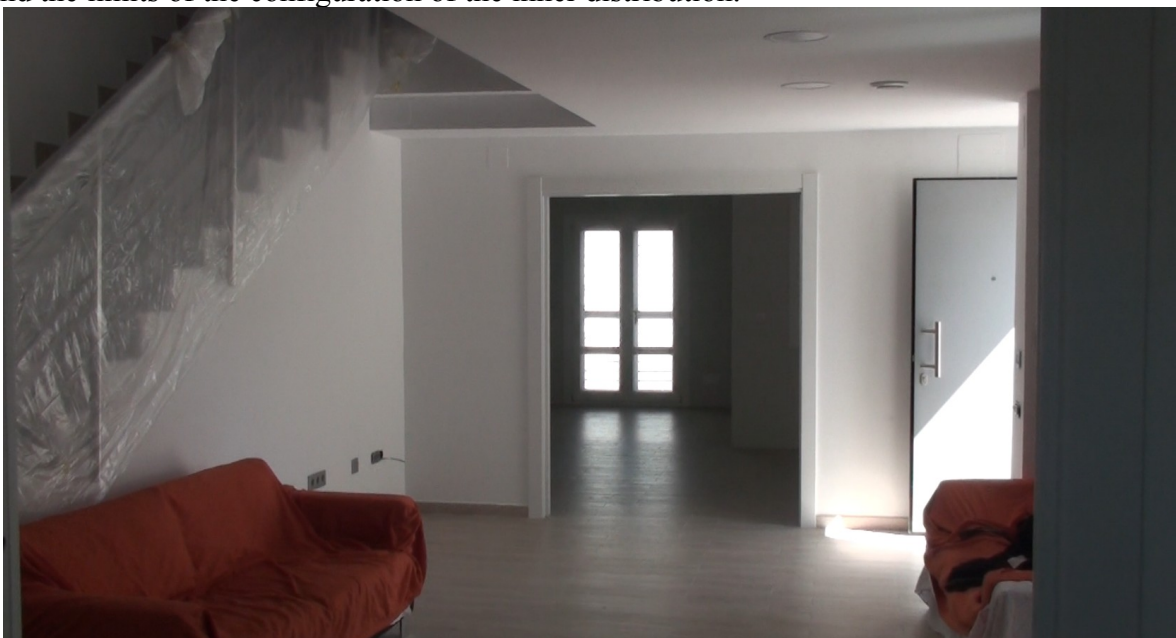
View from the living room to the kitchen
