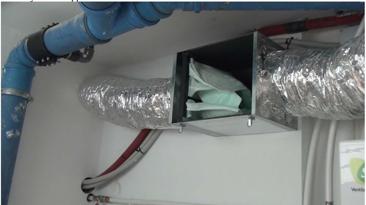
General air filter box which leads into the households
