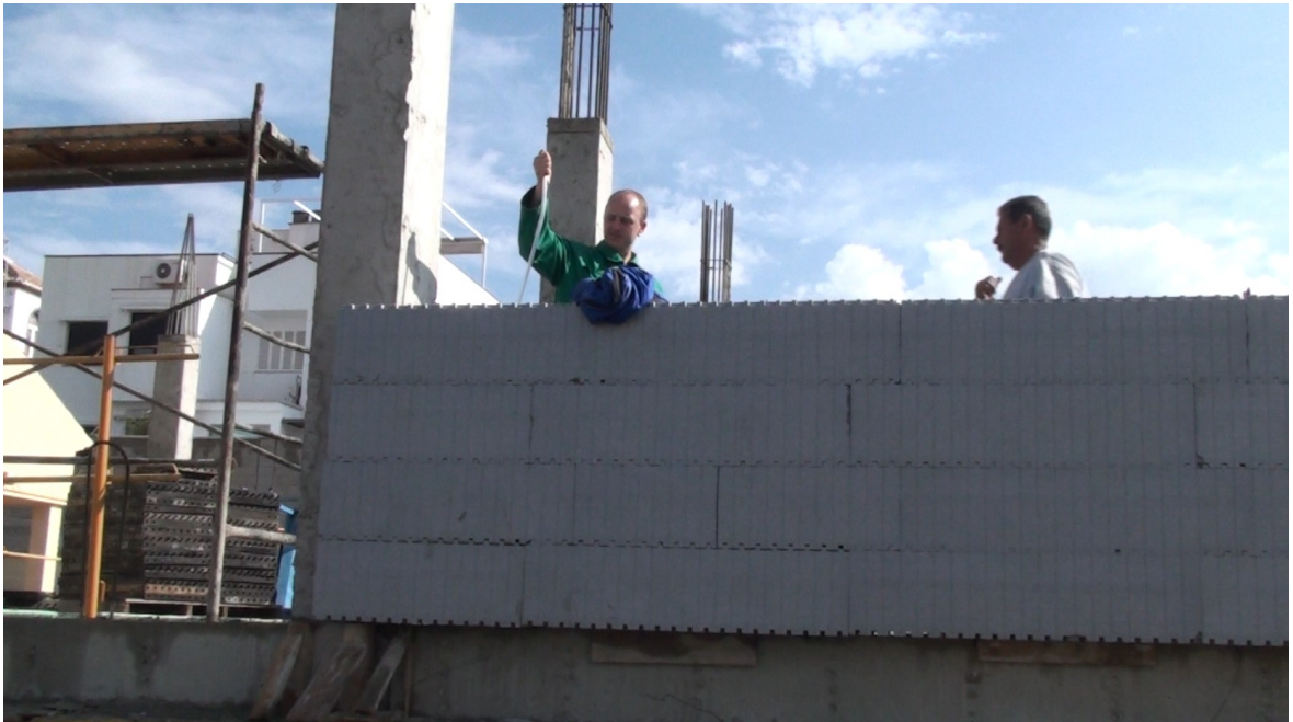
Day 1 19.04.2011 – Verification of level and vertical orientation of the walls
