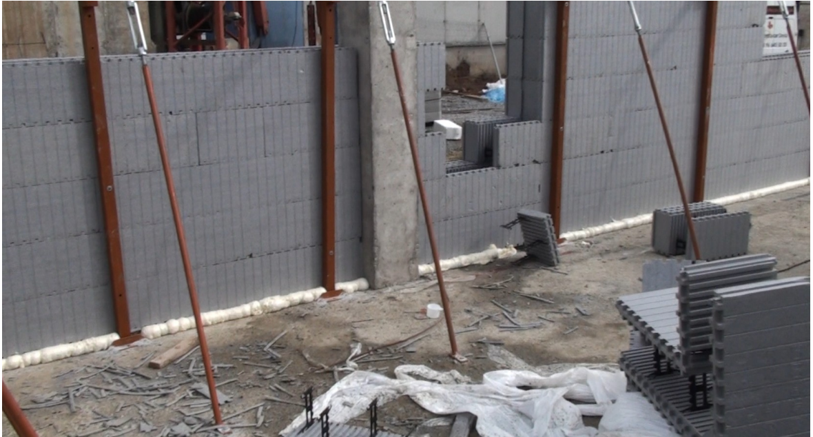
Day 1 19.04.2011 - Sealing of the lower part with pu-foam following the wall
