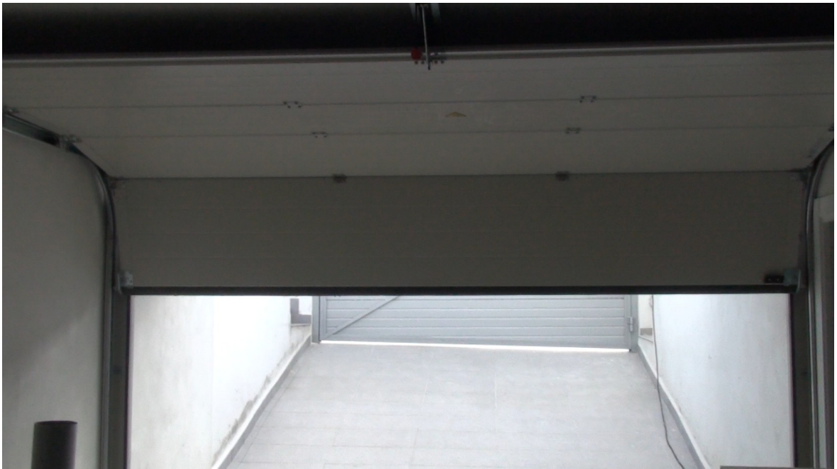
Sectional door Hörmann LPU40 with sandwich panel of 42 mm insulated with polyurethane
